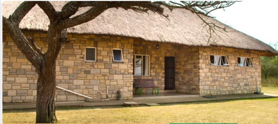
MSINSI ALBERT FALLS DAM
